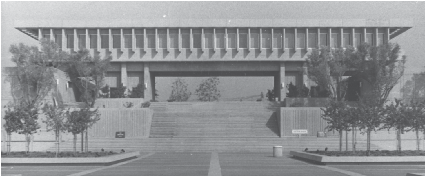
Stairway to pass underneath Central Complex (LADM) building.
