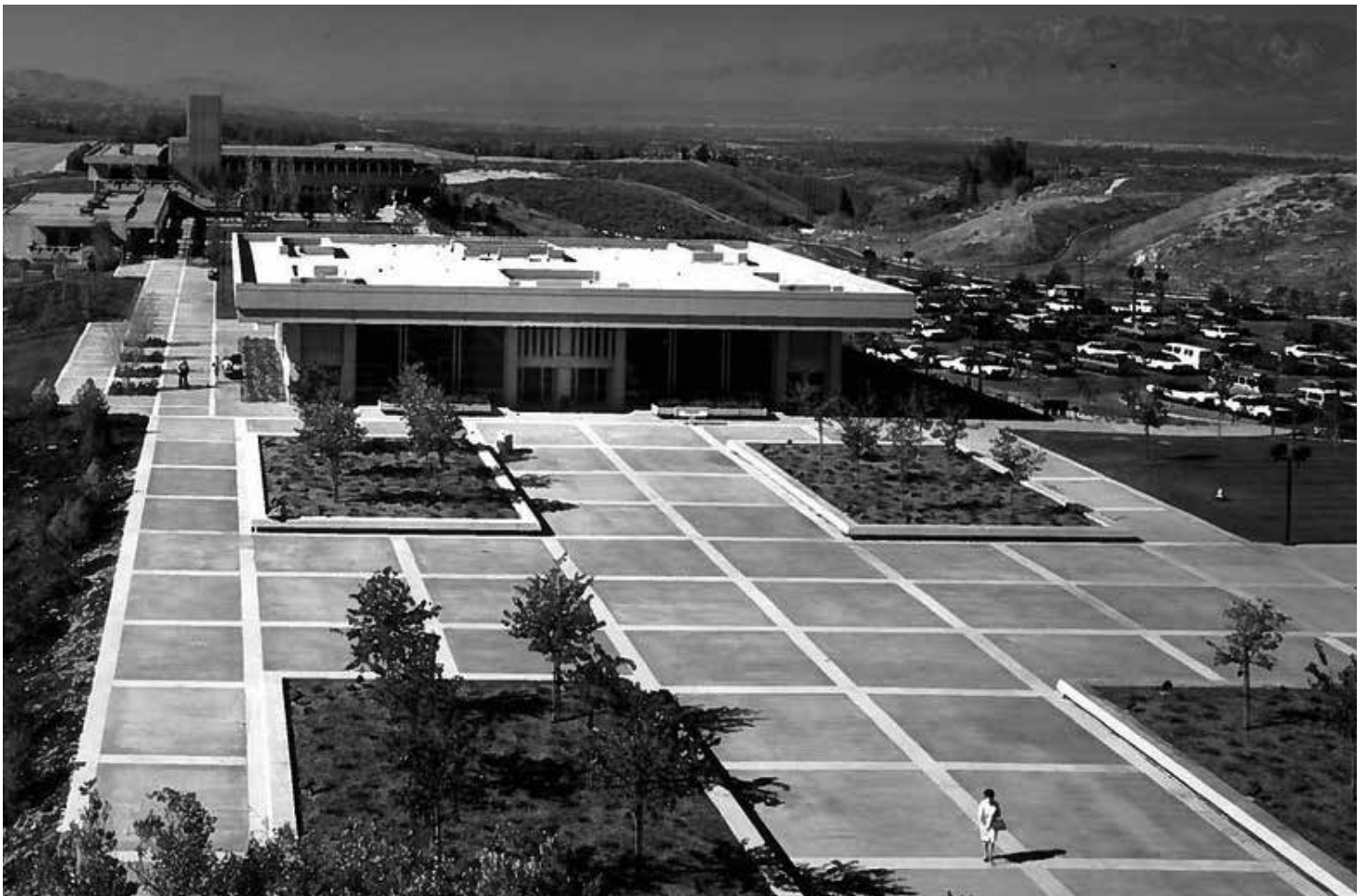
View of the library looking towards the clocktower.
