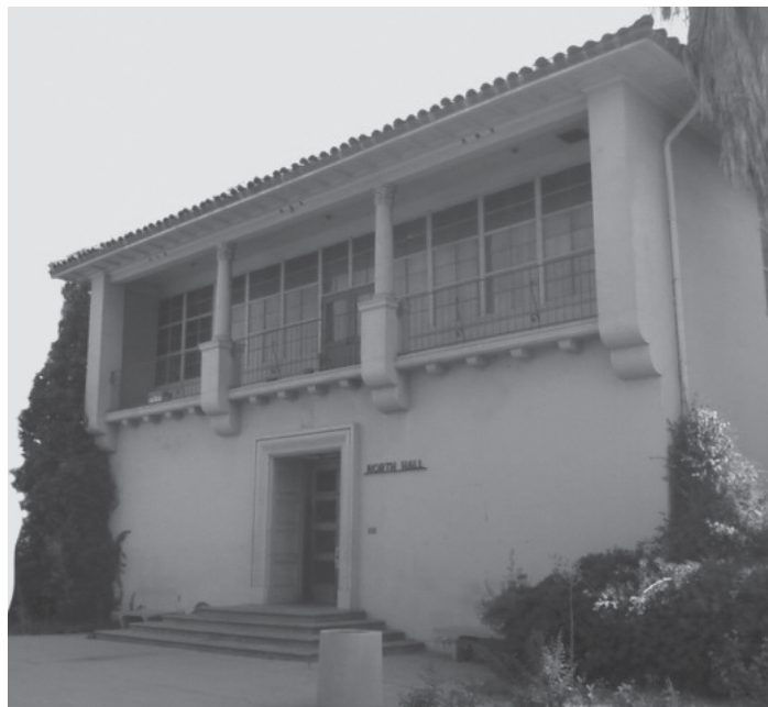
SBVC North Hall building.
