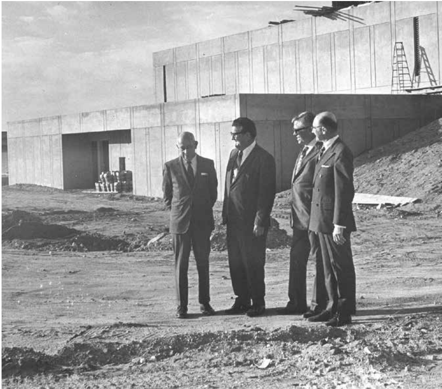
Lester Finklestein, Foster Davidoff and gentlemen at the construction site.
