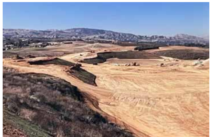
Land grading for the CHC campus.
