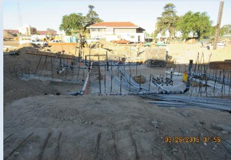
Segment B - Installation of Waste Piping and Electrical Conduits
