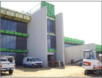
In the Learning Resource Center (LRC), painting, glazing and finishing touches (trim, light fixtures) were being finalized throughout May and June. Elevator installation preceded furniture delivery and exterior concrete walkways have been installed.
