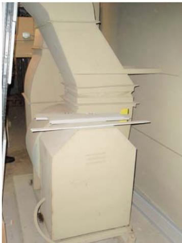
Mechanical room 243 serving biology labs have two 7.5HP and 5HP multizone units with economizer and VFDs on each supply fans, and have four 1/2HP exhaust fans, one 1HP exhaust fan, and one 7.5 HP vacuum blower. This mechanical room has also one 4.5kW, 58 gallons electric water heater with domestic hot water circulation pump.
