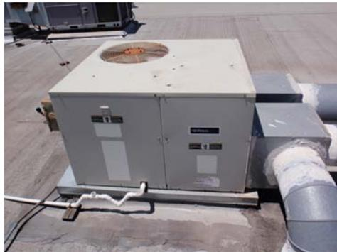
Heating/Cooling: In the building there is one multizone chilled water (240 MBH), duct furnace (600 MBH) unit with 7.5 HP supply fan motor on VFD. Chilled water is provided from chilled water loop connected to central plants. Total installed cooling capacity for the building is calculated as 45 tons (350 ft<sup>2</sup>/ton). Total installed heating capacity for the building is estimated at 300 MBH.
