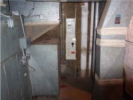
Mechanical room 227 has one 7,000 CFM multizone unit with economizer and VFD on supply fan.
