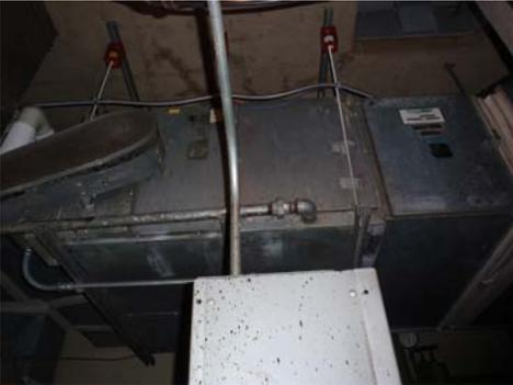
There are multiple exhaust fans in rest rooms and in labs. Laboratories have multiple exhaust fans. The relays of exhaust fans are being wired in to the Siemens APOGEE controller and during the time of this energy audit, they were not wired for LADM building. The exhaust fans on laboratories are reported to be scheduled based on instructor's requests in control system.
