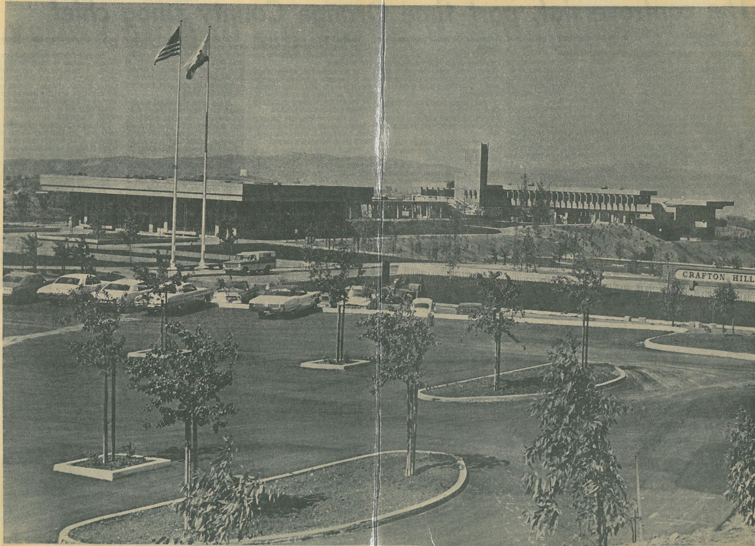
The new Crafton Hills College, which will open next month, sits on a hill above the Yucaipa Valley. (Staff photos by Darrell Santschi)
