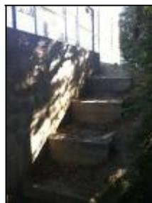
19. Steep, un-cleaned steps are being covered with loose gravel, leading to potential slips and falls.
