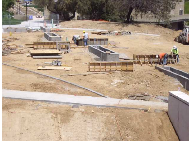
Grading is completed and further landscape work in progress.
