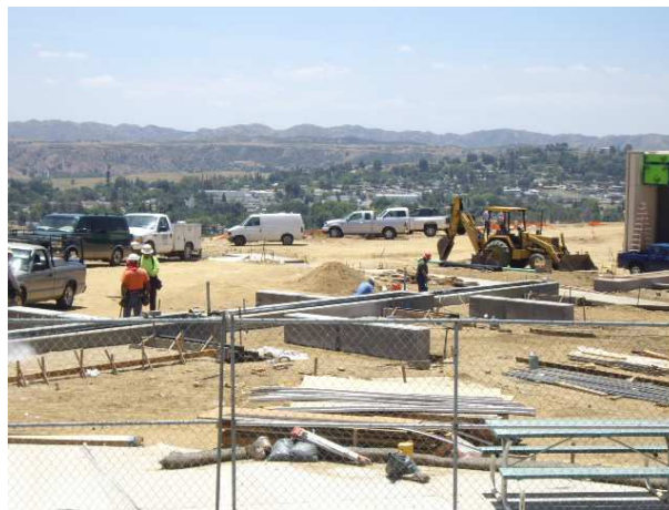
Walkways and planters in progress.
